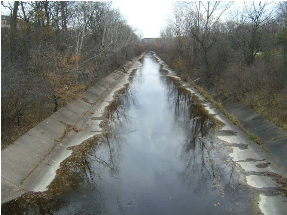
FIGURE 2 Concrete Lining in Underwood Creek
