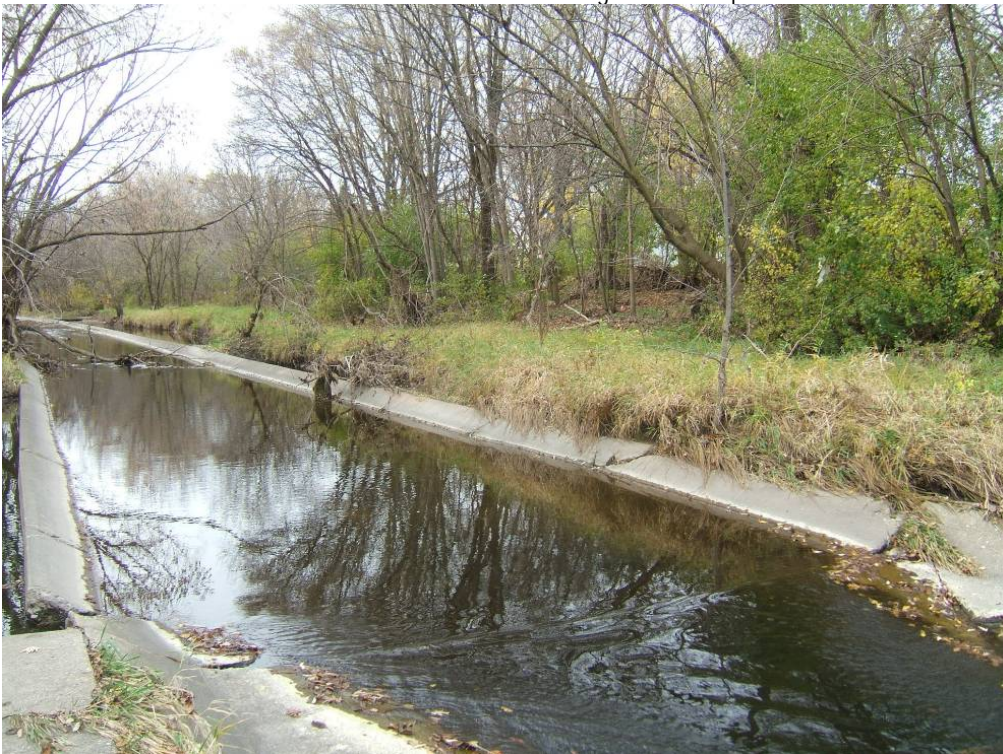
FIGURE 4 Underwood Creek Concrete-Lined Low Flow Channel with Vegetated Floodplain
