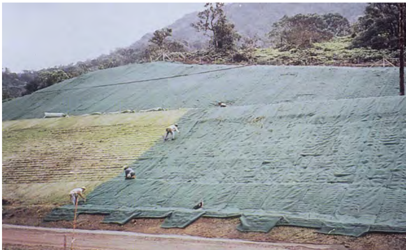
Figure 3-1: Geotextiles used for stabilizing a hillside
