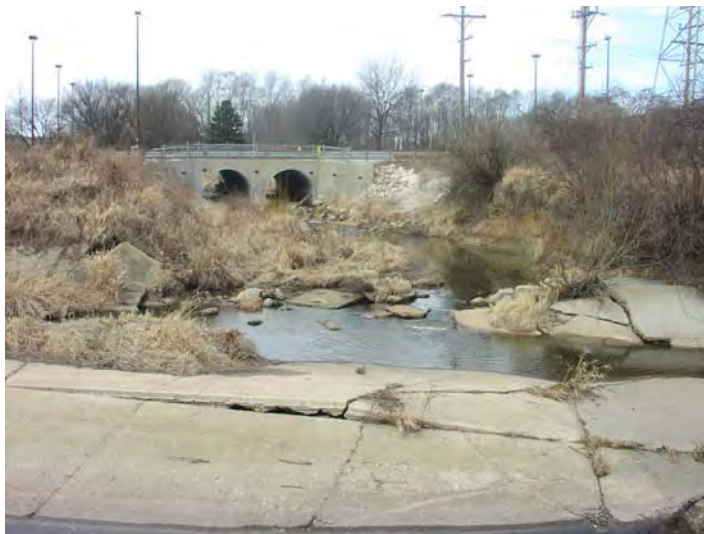
Before: Failing concrete streambank, downstream of UC-03
