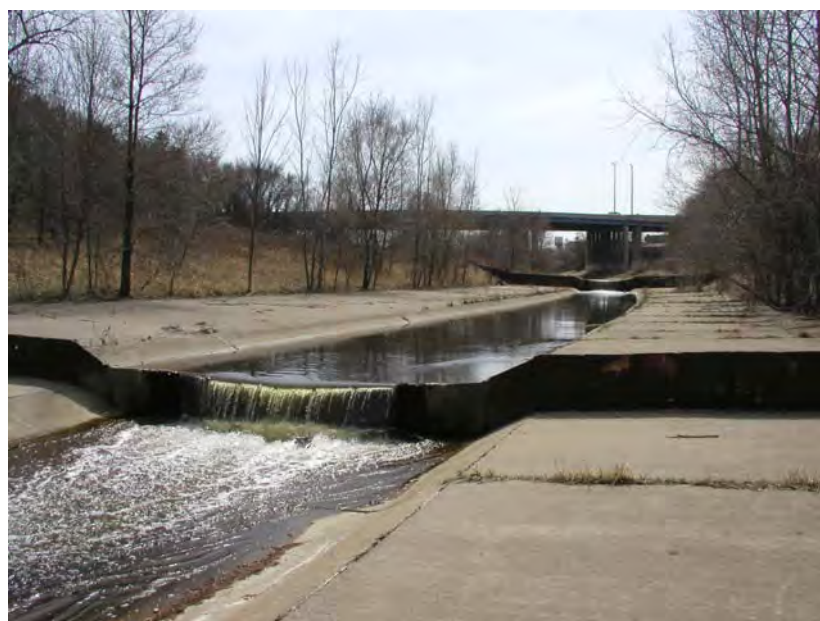
Underwood Creek, concrete lined and straightened channel
