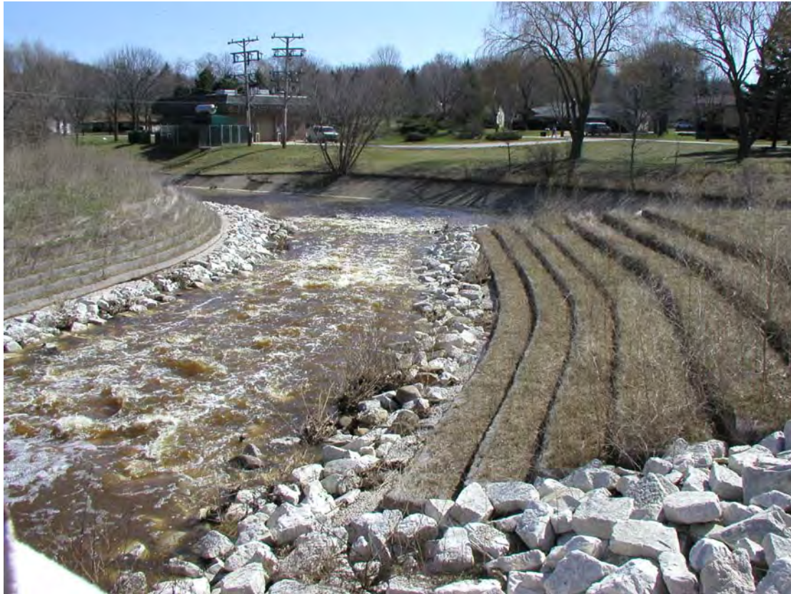
Underwood Creek, bioengineered channel.
